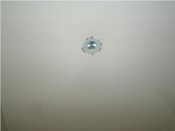
Damage to ceiling around light fitting
