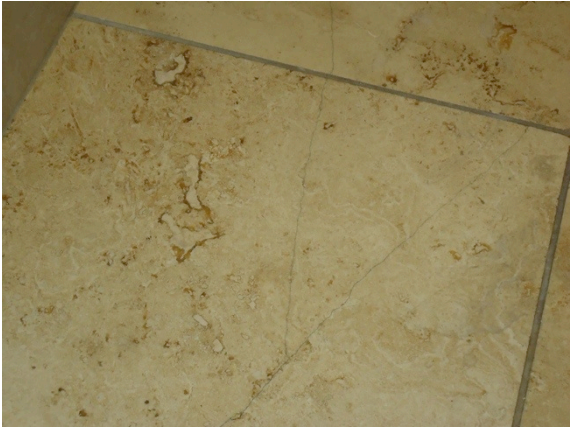
Example of cracked floor tiles
