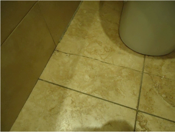
Example of cracked floor tiles
