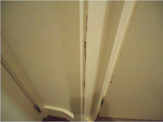
Cracking to exterior doorframe
